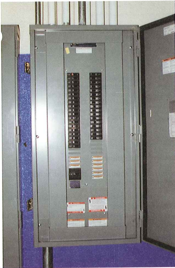
Figure 33 ♦ Typical panelboard.
