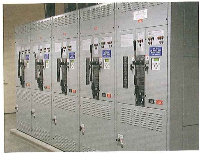
Figure 2 ♦ Typical low-voltage, metal-clad switchgear.
